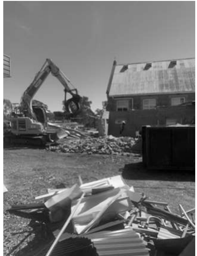
Demolition prior to re-building
