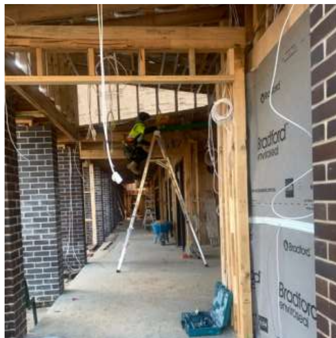
Work in progress at St Augustine's (See article page 12)
